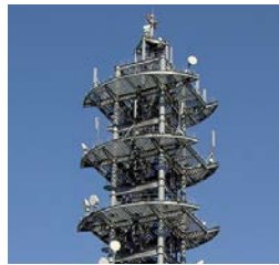
Large-zone base station that secures communications in densely populated areas in times of disaster
