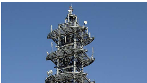
Large-zone base station that secures communications in densely populated areas in times of disaster
