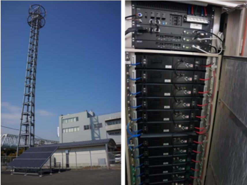
Solar panel and base station (left photo) and green electricity controller (top shelf) and high-capacity, rechargeable battery.
