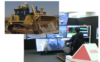
Remote operation of construction equipment, etc.
