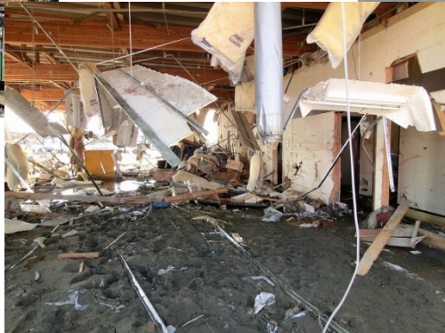
docomo Shop (Ishinomaki-Higashi, Miyagi: Interior)
