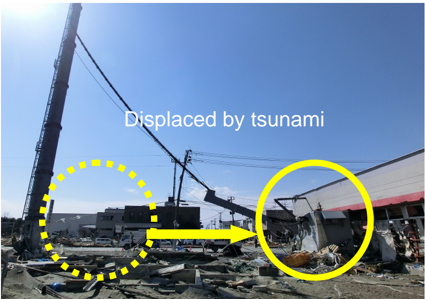
3. Base station facility (Ishinomaki-Midori-cho, Miyagi)
