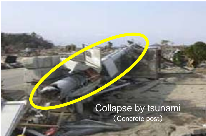
1. Base station facility (Matsuhima-Nobiru, Miyagi)
