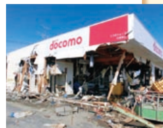
Ishinomaki East docomo Shop (Miyagi Pref.)
