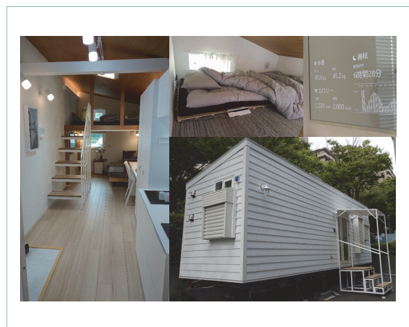
Figure 1 Exterior and interior views of IoT Smart Home
