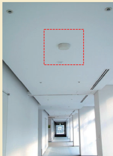
Photo 2 Indoor antenna installed in hallway
