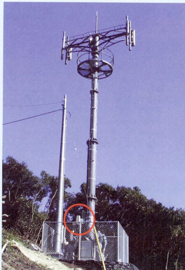
図2 マイクロBSの設置例 Figure 2 Example of Micro BS Setting Up.
